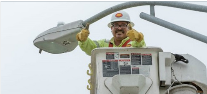
Installers add smart controllers to streetlights. These can manage lighting and communicate with nearby smart city sensors.
